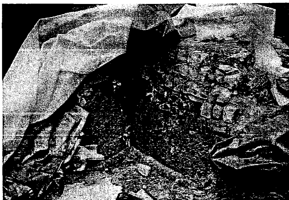
Photograph 11 South west corner of room II. As in the photograph above, areas covered by transparent plastic sheet appear to support more organic growth than those covered in opaque black plastic
